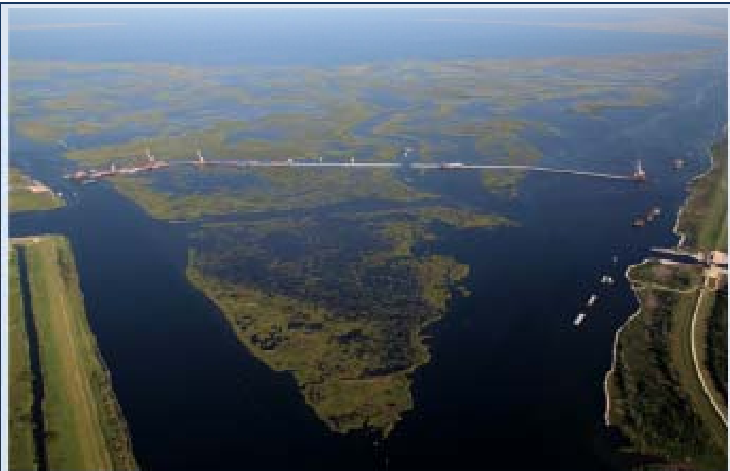
Figure 4. Aerial view of the partially-completed surge barrier across the MRGO-GIWW tunnel.
